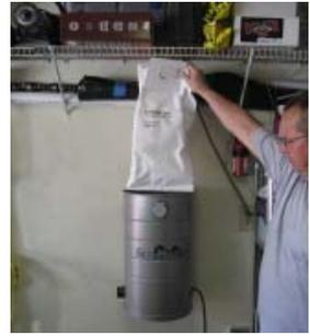
**Fig. 1** You will need to be able to remove the filter bag from the top of the unit. Be sure to leave enough room when mounting.
