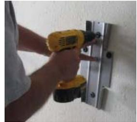
**Fig. 2** Mount the wall bracket.
